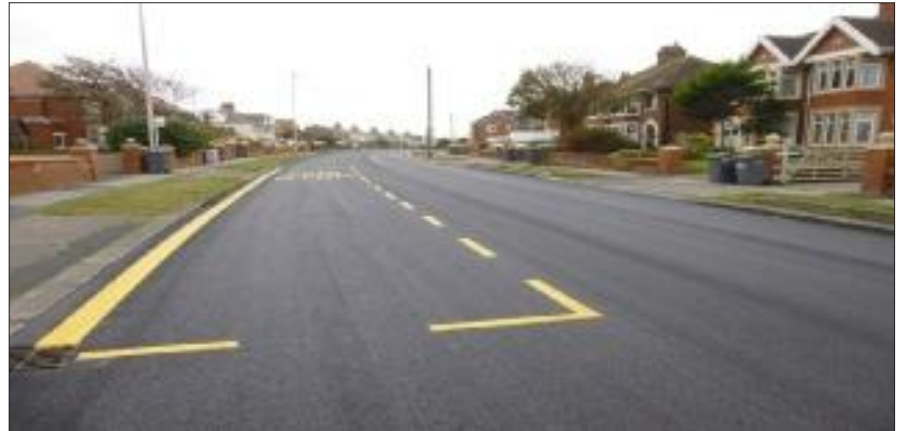
Blackpool, local roads treated with Rhinophalt preservation and new road-markings
